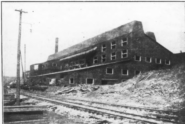
SMELTER AND CONVERTER BUILDING, CERRO DE PASCO
