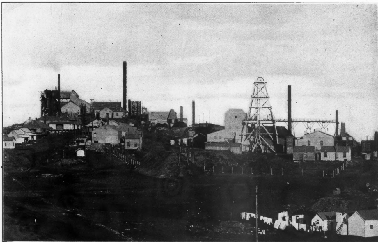
SURFACE PLANT, KALGURLIE GOLD MINES, LTD.
