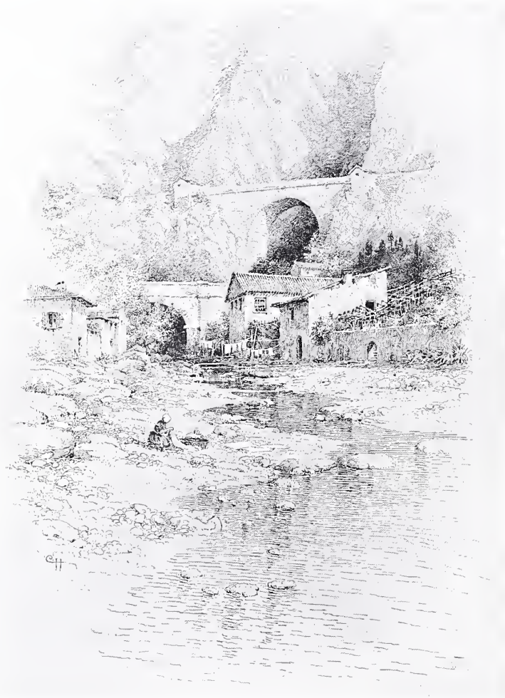
THE FRONTIER BRIDGE BETWEEN FRANCE AND ITALY, NEAR MENTONE.
