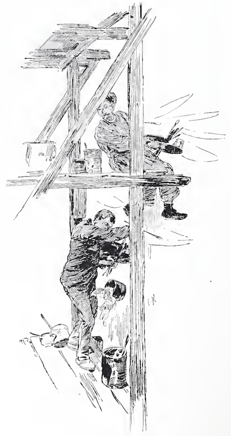
AT WORK ON TWO STOREYS.
