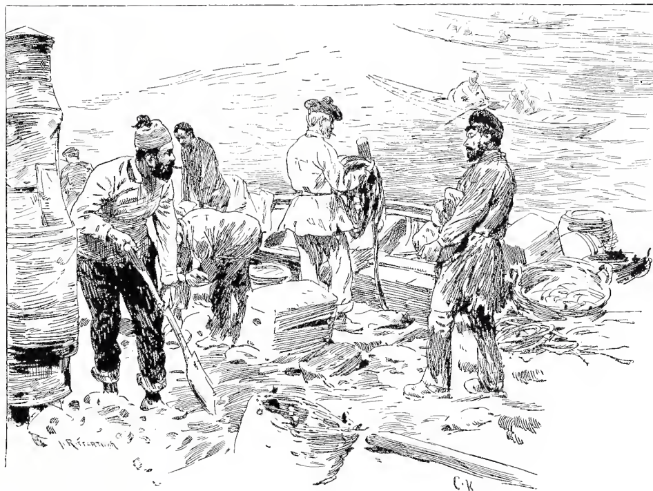
EXCAVATING FOR THE WATER.
