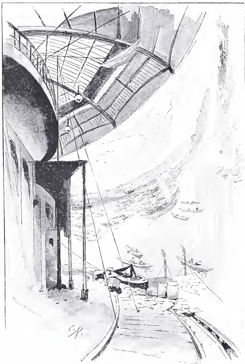
THE WORK IN PROGRESS, SEEN FROM BELOW.
