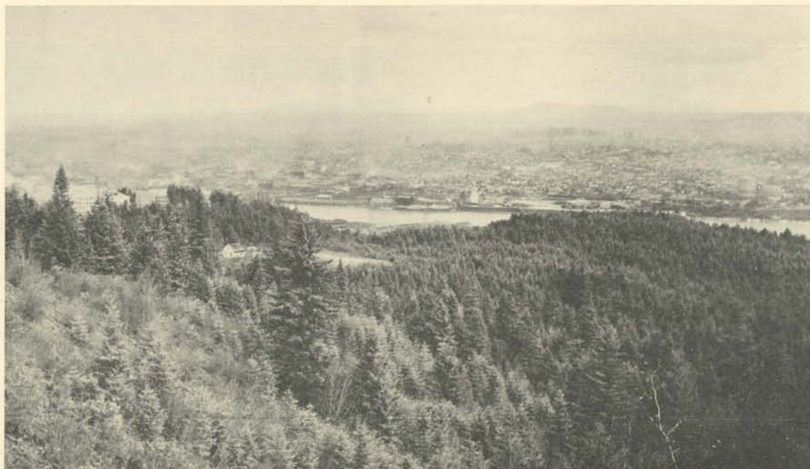
THE SITE OF THE NEW VETERAN'S HOSPITAL
