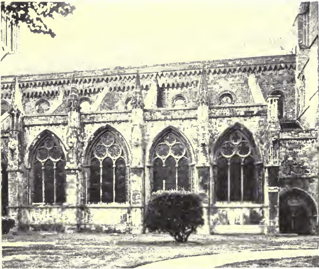
EXTERIOR OF THE NORTH SIDE OF NAVE
