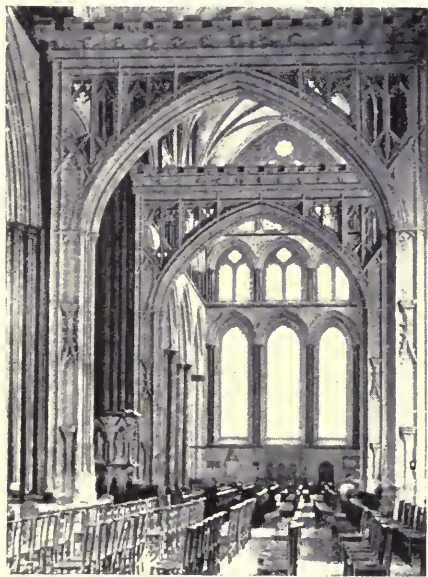
XVTH CENTURY STONE GIRDERS IN TRANSEPT
