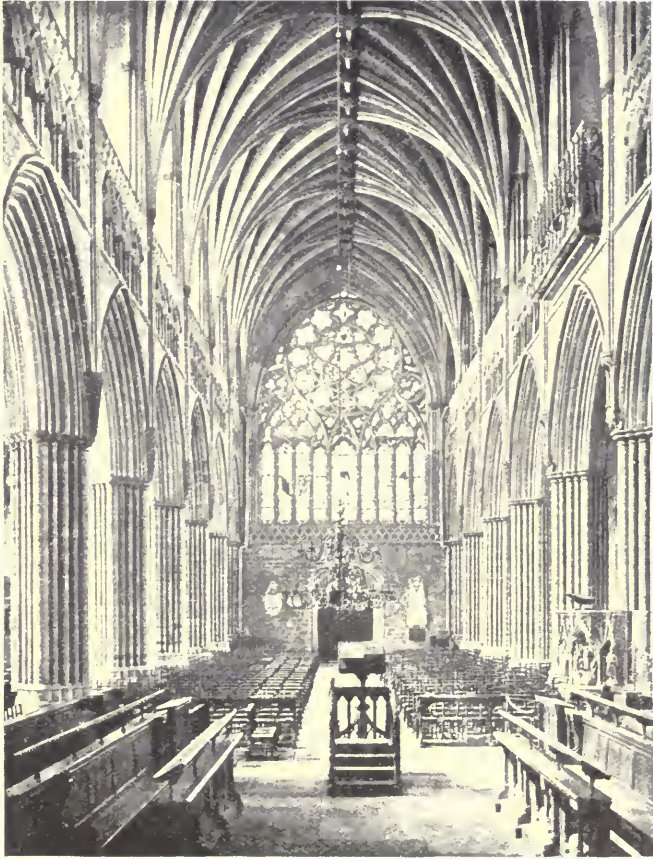
THE NAVAL, LOOKING WEST
