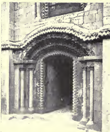
THE SOUTH TRANSEPT DOOR
