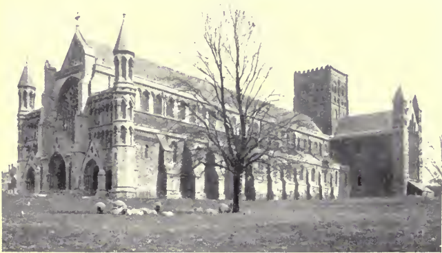
FROM THE SOUTH-WEST, SHOWING THE NEW WEST FRONT
