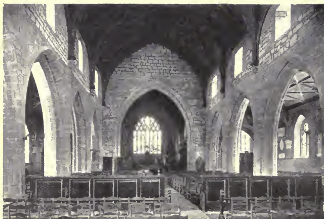
THE NAVE, LOOKING EAST
