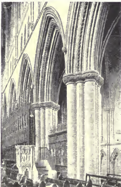
PIERS ON THE NORTH SIDE OF THE CHOIR
