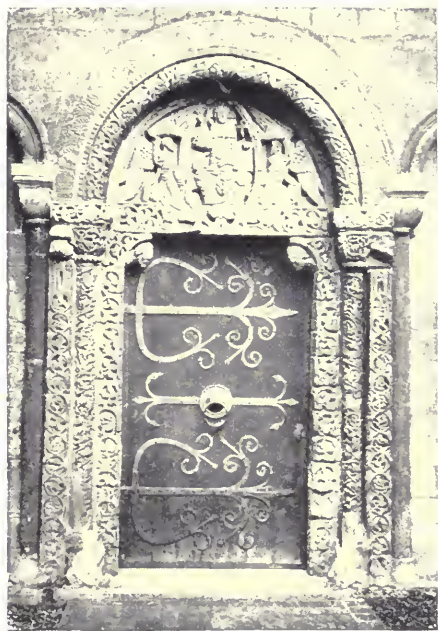
WESTERN PROCESSIONAL DOORWAY
