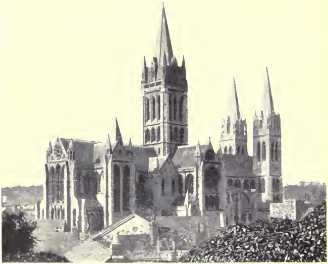
GENERAL VIEW FROM THE NORTH-EAST
