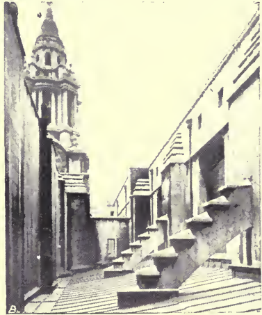
THE FLYING BUTTRESSES AND SCREEN WALL
