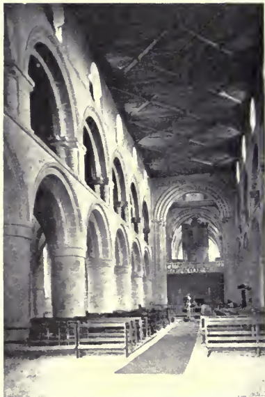
THE NAVE, LOOKING EAST
