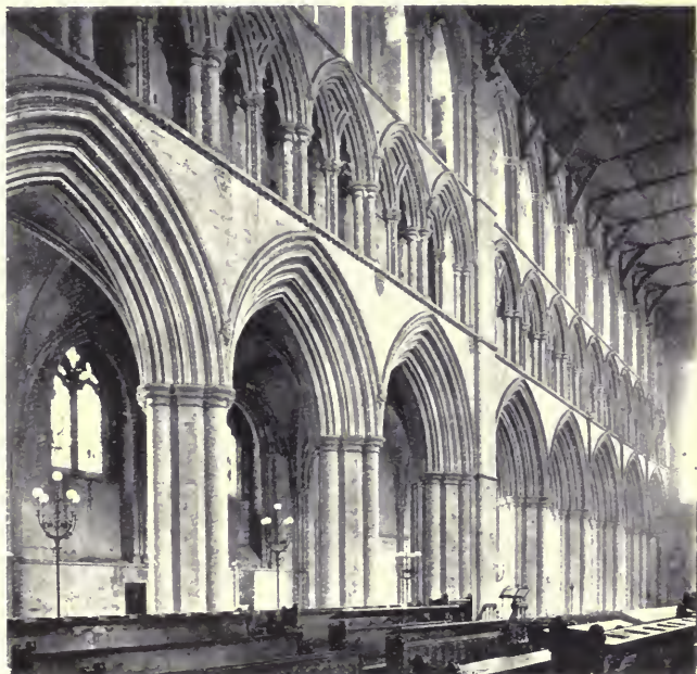
THE SOUTH ARCADE, LOOKING WEST
