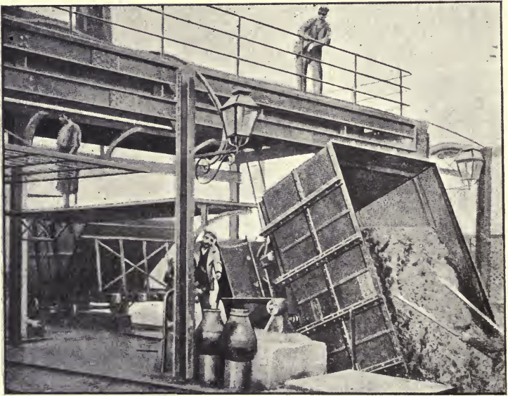
FIG. 195.—Systematic levigation of the bagasse. Perichon's process as used in Egypt (CAIL).
