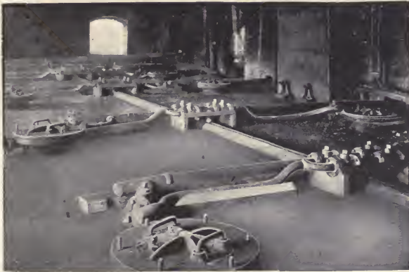
FIG. 226.—Covers of animal charcoal filters with piping.
