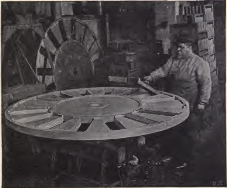
FIG. 20.—Removing knife-holders from plate of beet-slicing machine.
