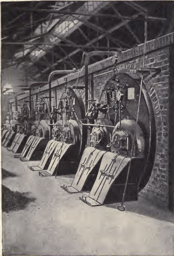
FIG. 102.—View of stoke-hole and boilers of Leopoldsdorf beet-sugar factory for providing steam for evaporation and concentration of juice.
