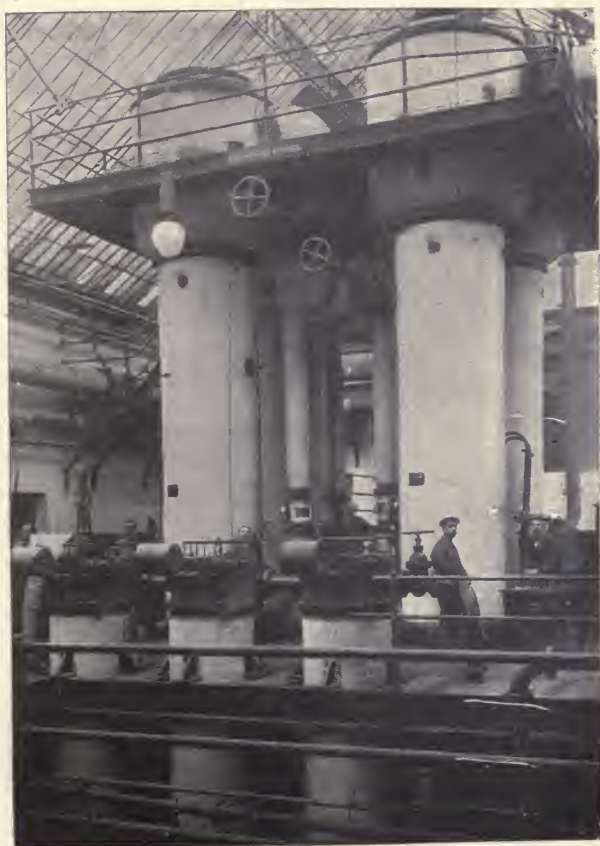
FIG. 223A.—Kestner quadruple effect. Tirlémont sugar refinery, Belgium.
