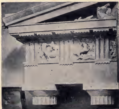
FIG. 27.—DORIC ORDER OF THE PARTHENON.
