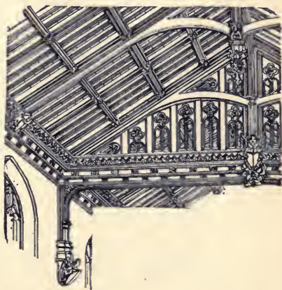
FIG. 138.—ROOF OF NAVE, ST. MARY'S, WESTONZOYLAND.
