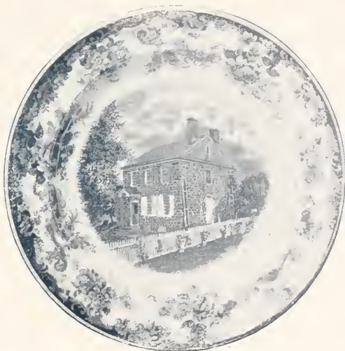
WASHINGTON'S HEADQUARTERS, 1777-78 Valley Forge, Pa.
