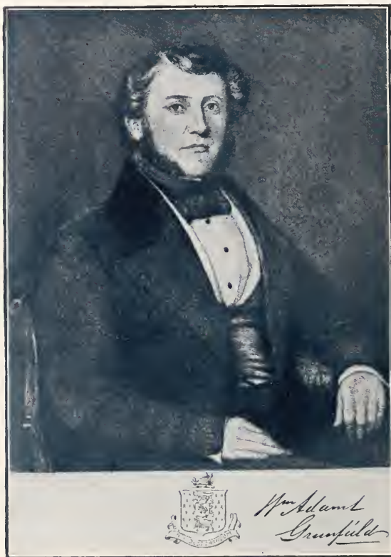
William Adams, of Tunstall and Greenfield.
