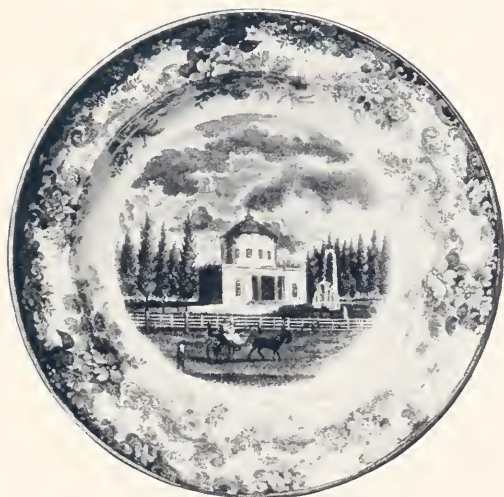
109 m. Water Works, Center Square, Philadelphia.
