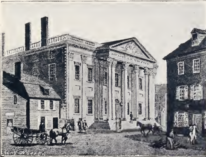
Bank of the United States. (Old print from which the Stubbs design was copied.)
