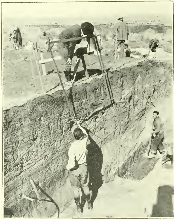
2. NEW TYPE "STRATAGRAPH" USED IN MAKING RAPID AND ACCURATE DIAGRAMS OF DEEP STRATA AT TULAMNIU.
