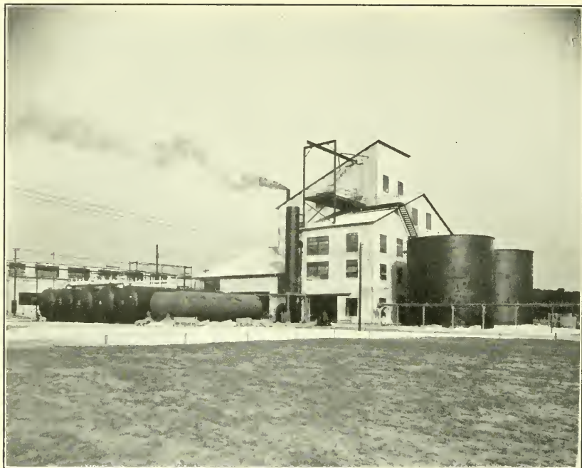
1. BROMINE AND ETHYLENE DIBROMIDE PLANT.
