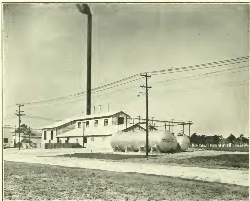
2. ETHYLENE PLANT AND POWER HOUSE.
