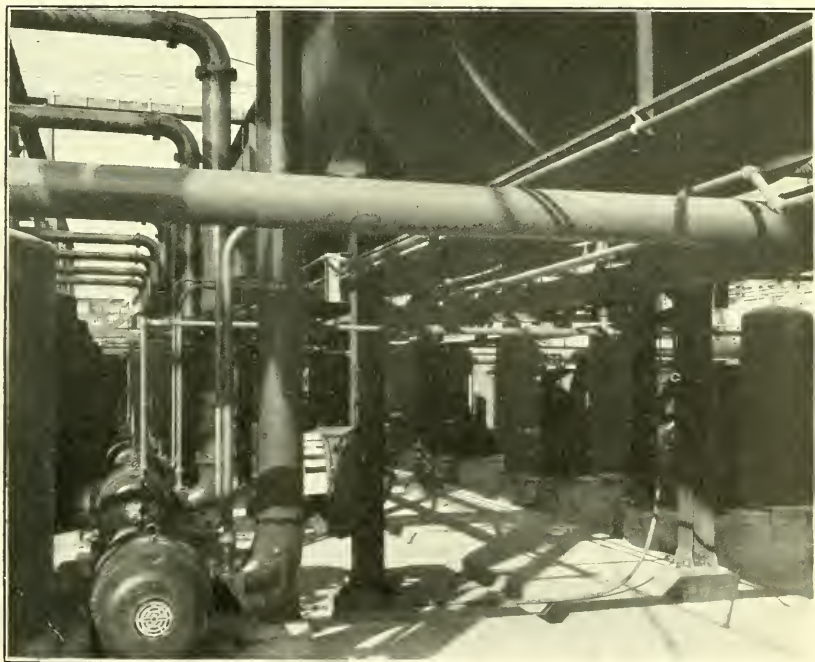
2. BATTERY OF PUMPS FOR CIRCULATING BROMINE ABSORPTION LIQUOR.
