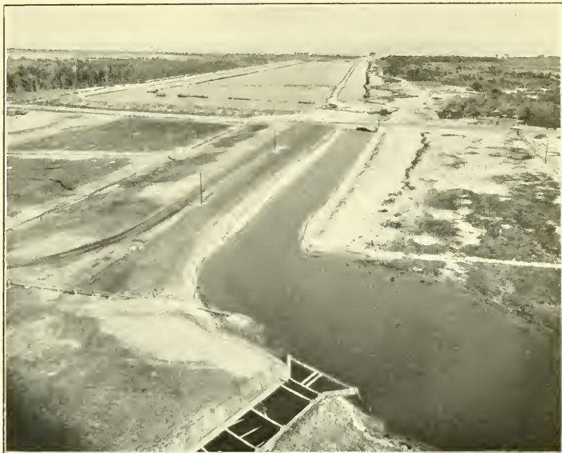
1. CANAL AND POND FOR PASSING SEA WATER TO BROMINE EXTRACTION PLANT.
