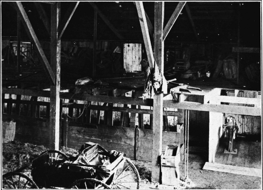
FIG. 2.—A STABLE THAT IS DIFFICULT AND EXPENSIVE TO KEEP CLEAN.
