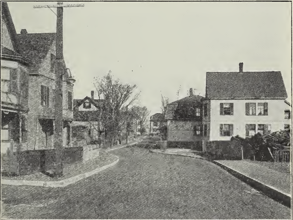
HINCKLEY STREET, AFTER ACCEPTANCE AND CONSTRUCTION
