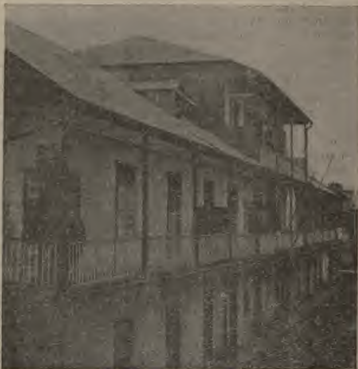
"STAR & HERALD" BUILDING, WHERE THE PAPER WAS FIRST PUBLISHED.
