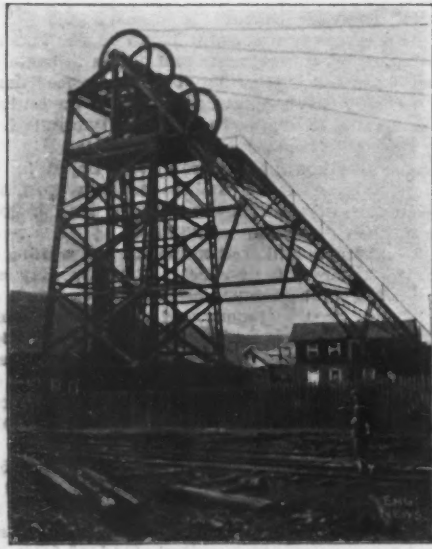
Fig. 1. Perspective View of Steel Head Frame for the Philadelphia & Reading Coal and Iron Mines, at Gilberton, Pa.
