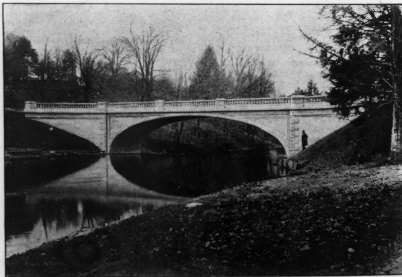
FIG. 2.—MELAN CONCRETE ARCH, WITH MOLDED CONCRETE FINISH, ON F. W. VANDERBILT'S GROUNDS, HYDE-PARK-ON-HUDSON.
