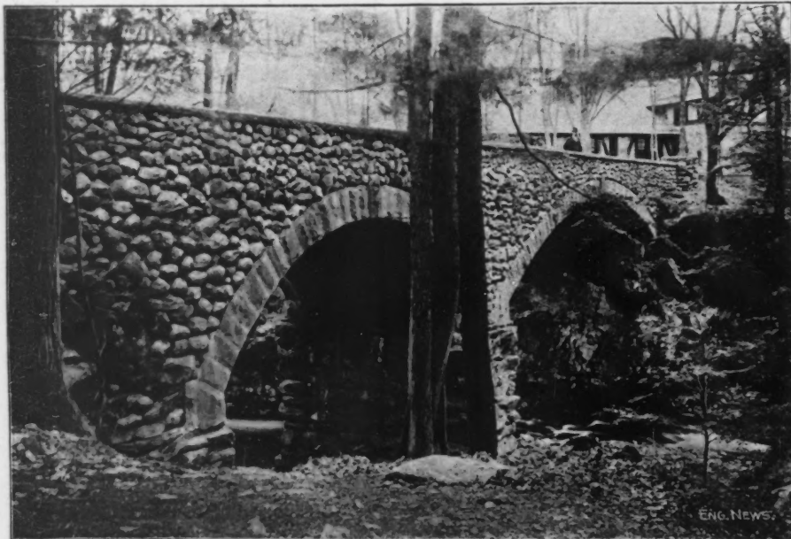
FIG. 1.—MELAN CONCRETE ARCH, WITH FIELD STONE FACING, ON GROUNDS OF FREDERICK W. VANDERBILT, HYDE-PARK-ON-HUDSON, N. Y.
