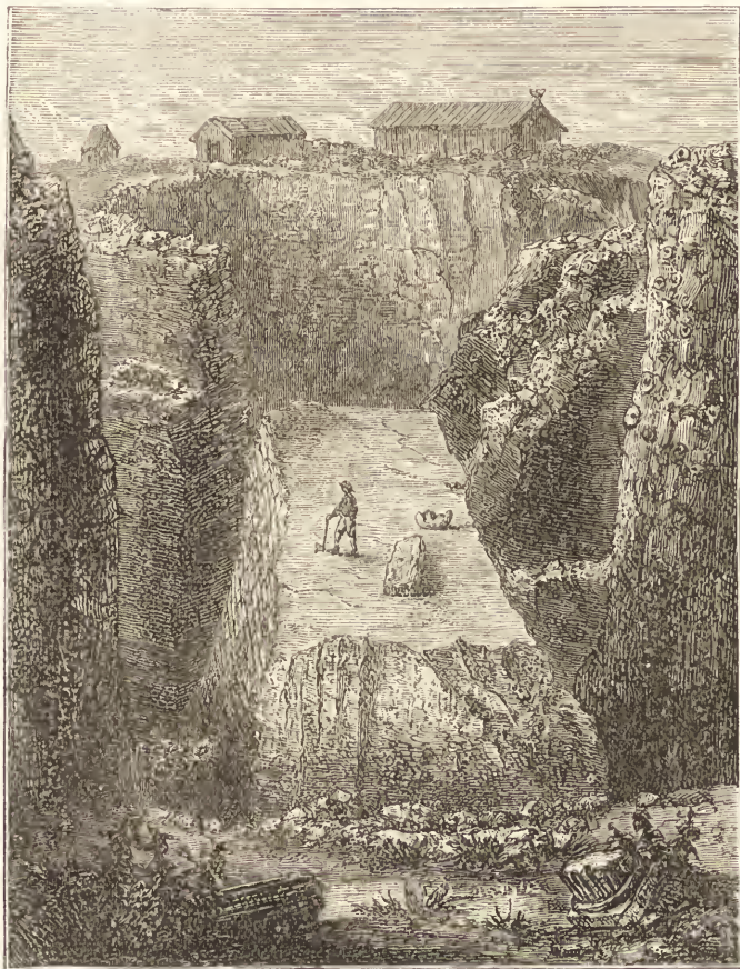
No. 3. The Great Tower of Ilium, seen from the S.E. The top is 8 m. (26 ft.) below the surface of the hill: the foundation is on the rock, 14 m. (46½ ft.) deep: the height of the Tower is 20 ft.
