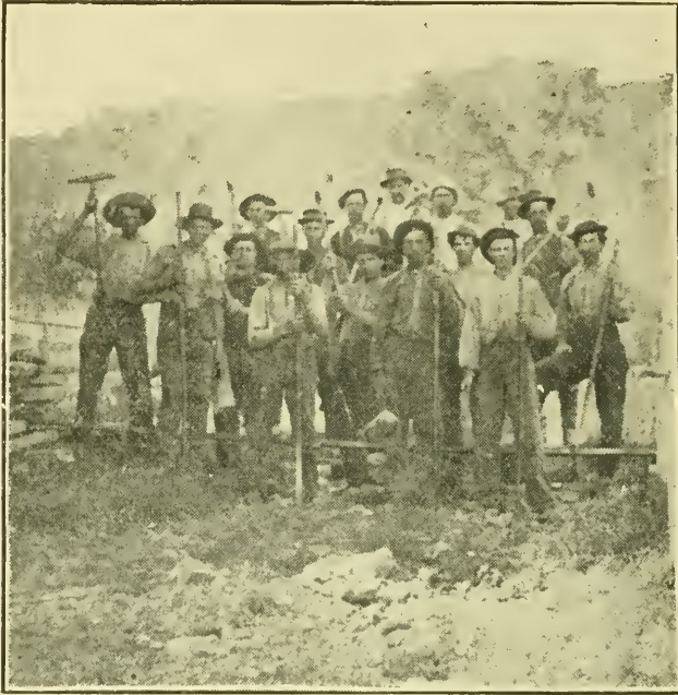
GRADING THE SUNBURY AND LEWISTOWN RAILROAD.
