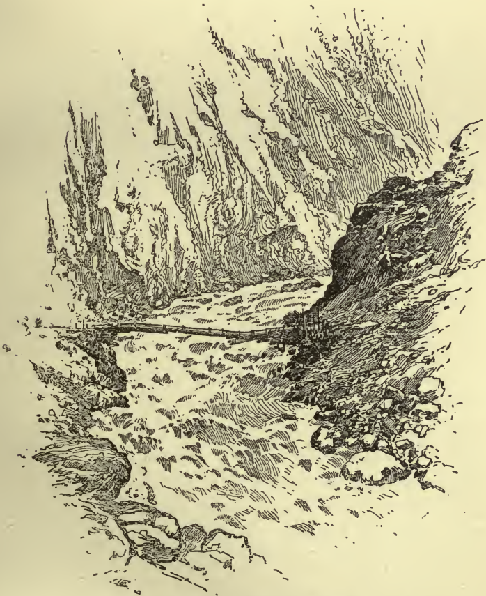
SHAITAN NARA, OR THE DEVIL'S BRIDGE. CANTILEVER BRIDGE OVER THE ASTOR RIVER.
