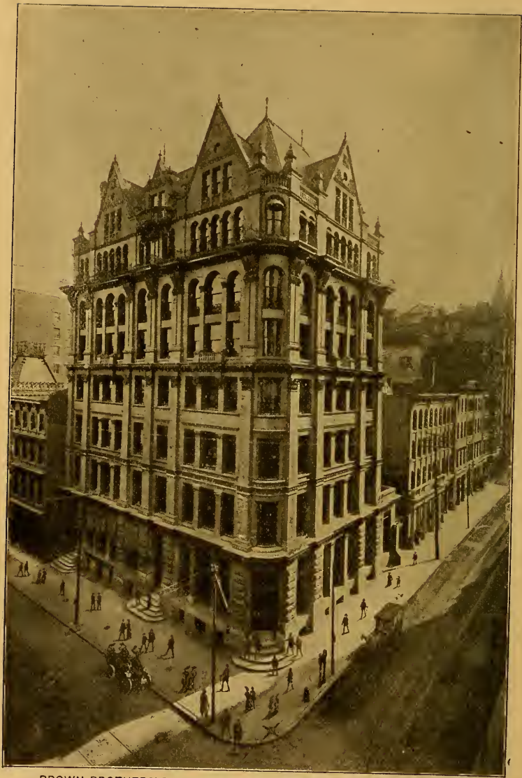
BROWN BROTHERS' BUILDING—Southwest Corner Fourth and Chestnut Streets.
