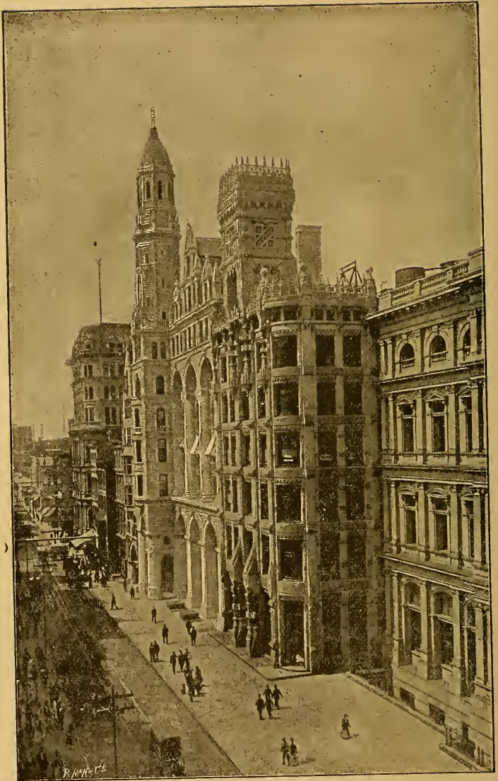
CHESTNUT STREET, LOOKING WEST FROM NINTH STREET.
