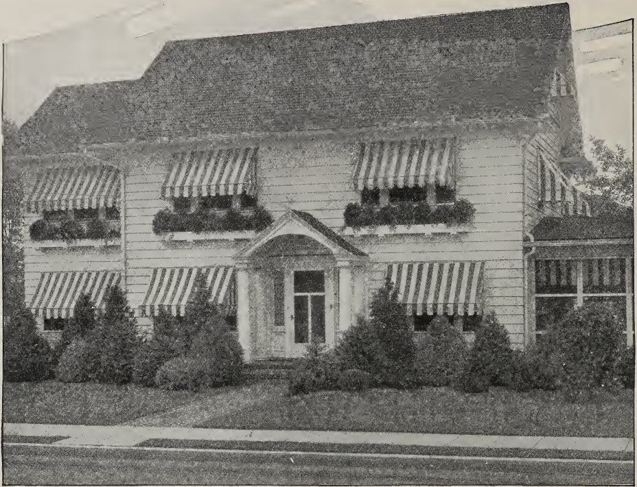
Foundation Planting of Juniper, Arbor Vitae and Spruce
