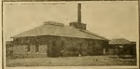
Water Works Plant
