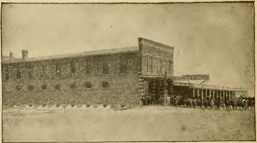
The John Becker Store, Belen
