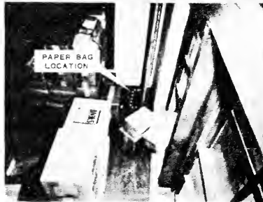
↑ SOUTHEAST CORNER OF SIXTH FLOOR. LOOKING EAST
