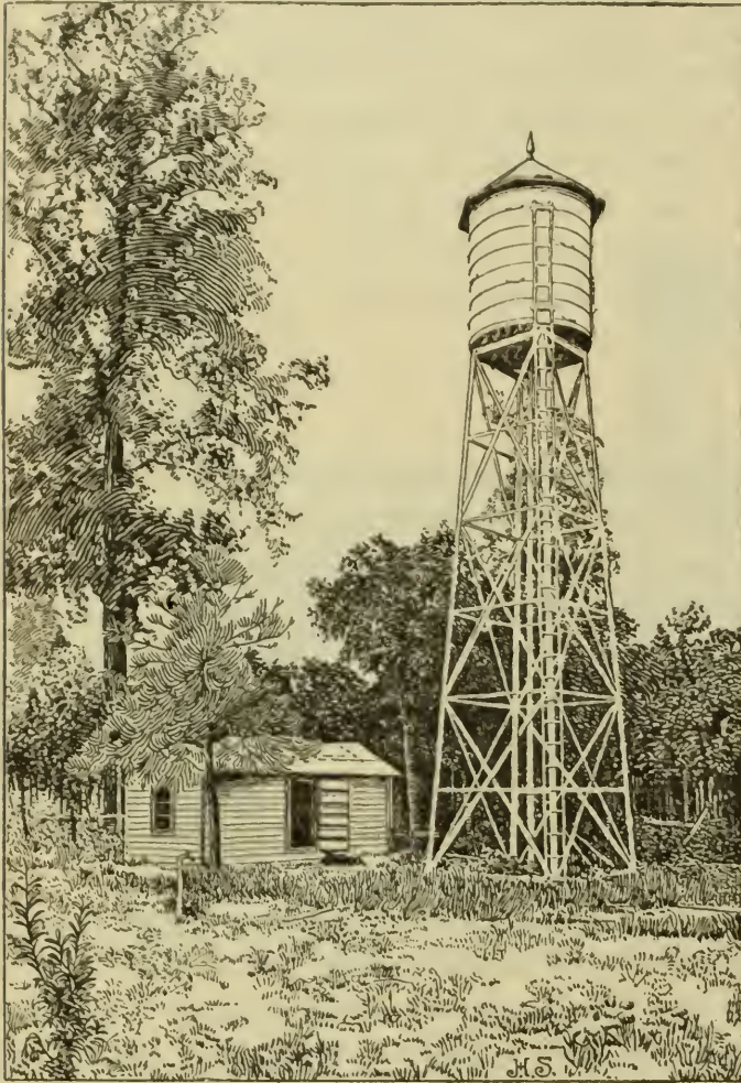
FIG. 20.—Tank and pump house for a home water supply.
