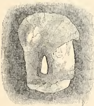
South Window, Interior
