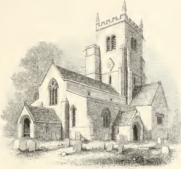
General View from the South-west.
