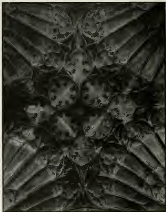
F. B. Gloucester: South Bay of East Cloister
