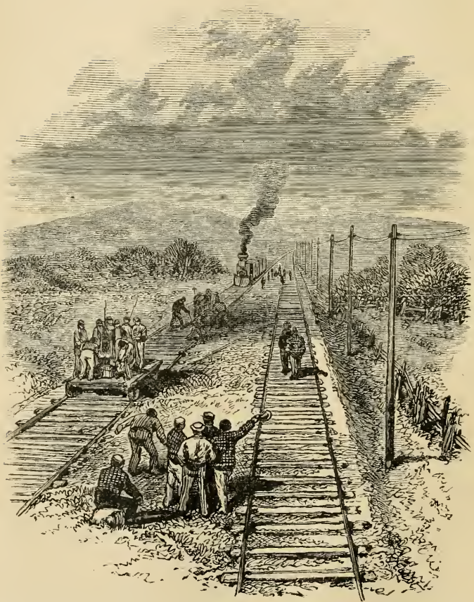
THE CONSTRUCTION GANG REPAIRING THE TRACKS UNDER PROTECTION OF THE MILITIA.
