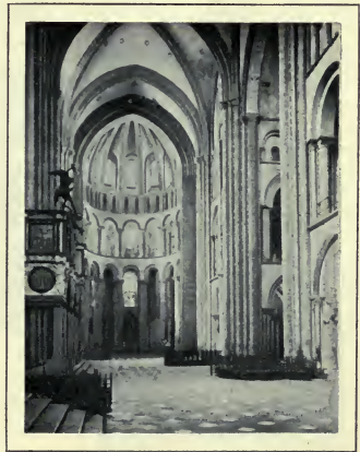
FIG. 5.—TRANSEPT OF CATHEDRAL (Eleventh Century). (Phot. Nels.)
