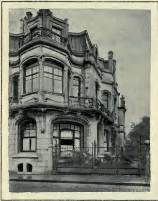
FIG. 536.—VICTOR HORTA. DETAIL OF THE FAÇADE OF THE HÔTEL AUBECQ (550, Avenue Louise, Brussels).
