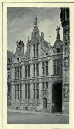
FIG. 267.—BRUGES. LAW COURTS. (Phot. Nels.)
