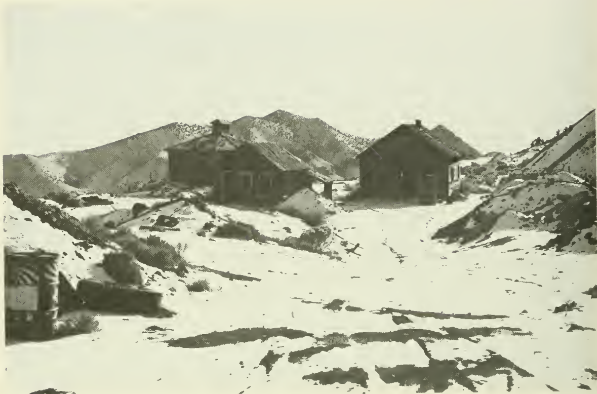
Fig. 28. Abandoned mine buildings and mine dump, Frisco, Beaver Co., Utah.
