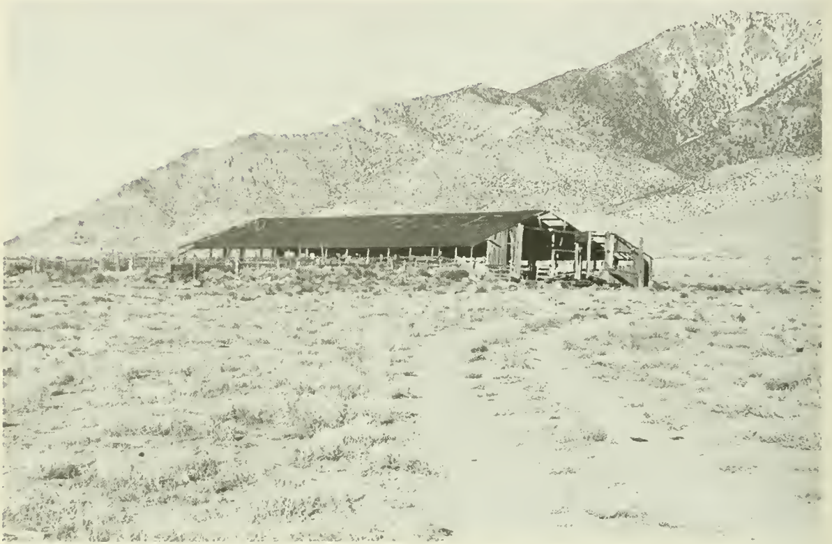
Fig. 5. Newhouse shearing sheds and corrals. As many as 200,000 head of sheep were reported to have been sheared here during a single year. Wah Wah Valley, Beaver Co., Utah.
