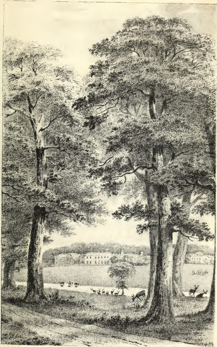
SOUTH WEST VIEW OF WOODS & ARCADE
