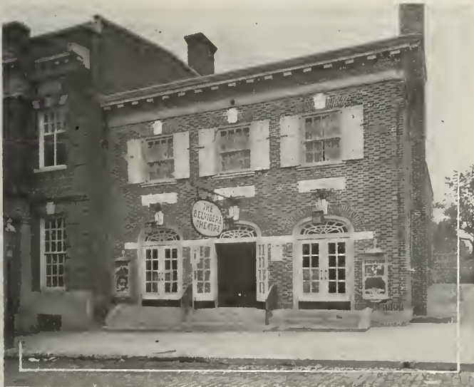
EXTERIOR OF THE BELVIDERE THEATRE
