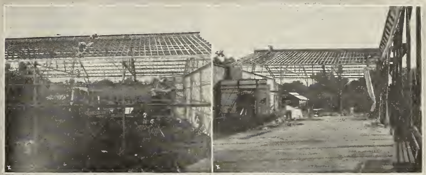
FINISHING THE FRAMEWORK
