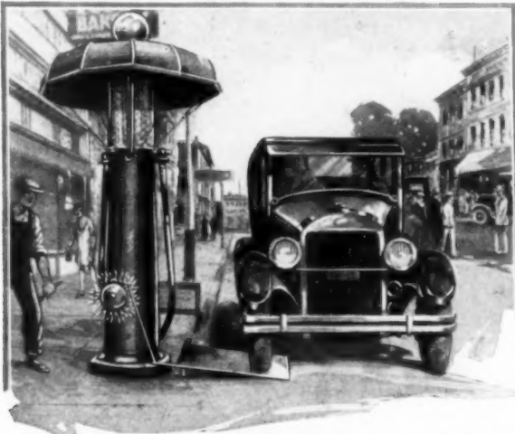
Gasoline Filling Pump with Umbrella Canopy, and Treadle by Which the Car Sounds Bell Signal for Service
