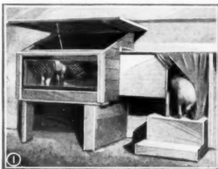
Comfortable Winter Quarters for Dogs Are Heated with Warm Air from the Basement; the Entrance Has Four Curtains to Keep Out the Cold Air
