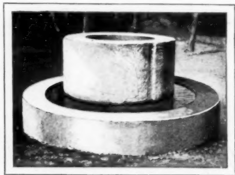
Circular Concrete Watering Trough for Hogs Cannot Be Overturned
