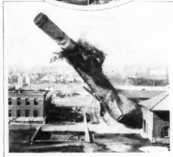
Big Chimney Splitting Just as It Fell; Cutting Away the Bricks for Temporary Timbers That Were Burned, and Stack an Instant before Final Collapse
