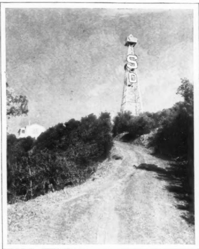
Powerful Airplane Beacon and Tower with Identifying Letters; the Light Can Be Seen for More than 100 Miles
