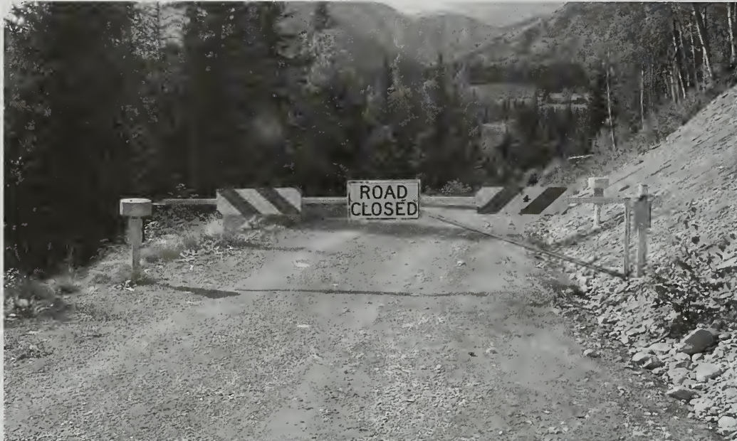
Rabbit Creek Road Seward Ranger District (Maintenance Level 1)
