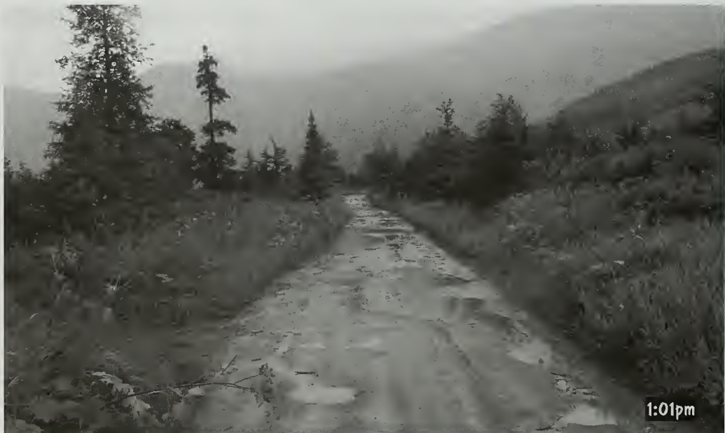
Upper Palmer Creek Road Seward Ranger District (Maintenance Level 2)
