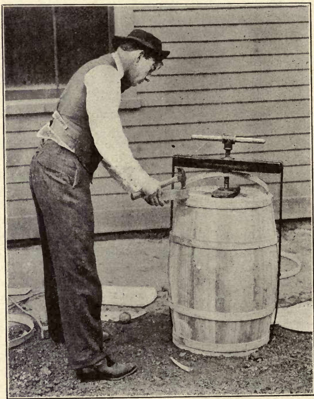
HEADING UP THE BARREL—SCREW PRESS
