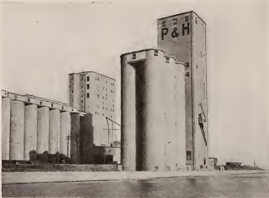
FIRST UNIT OF PARRISH-HEIMBECKER ELEVATOR, NOW IN OPERATION
