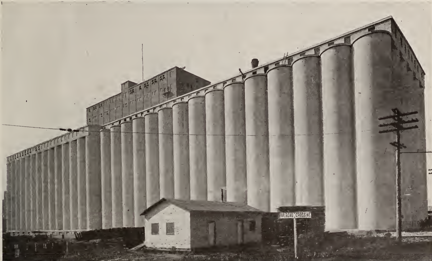
NEW ANNEX OF THE NORTHERN CENTRAL ELEVATOR AT BALTIMORE, MD.
