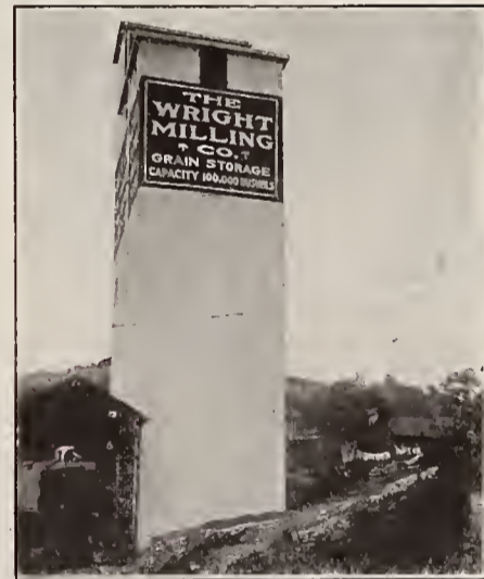
Reinforced Concrete Grain Elevator erected by us for The Wright Milling Co., Bluefield, W. Va.
