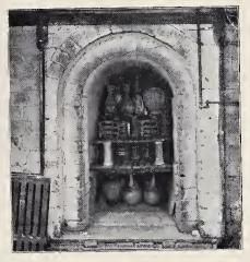
An Enamel Kiln.—This kiln or "glost-oven" is used for firing on enamel colours which are painted over the glaze. The heat is about a cherry red, sufficient to melt the flux mixed with the colours. There is no necessity to have the articles put in seggars or five-clay boxes, as no smoke or flame comes in contact with the work
