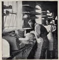
A Plate-maker at work.—The wheel is called a "jigger," and the mould is revolved upon it. The potter beats out a pancake of clay and dexterously throws it upon the mould, and after pressing it with a moist sponge he takes a tool called a profile and shapes the back of the plate by pressing the clay against the mould, which causes the foot to risc.
