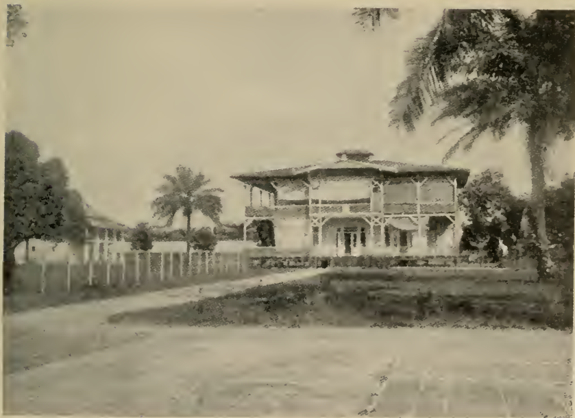
COURT HOUSE AT DUALA.
