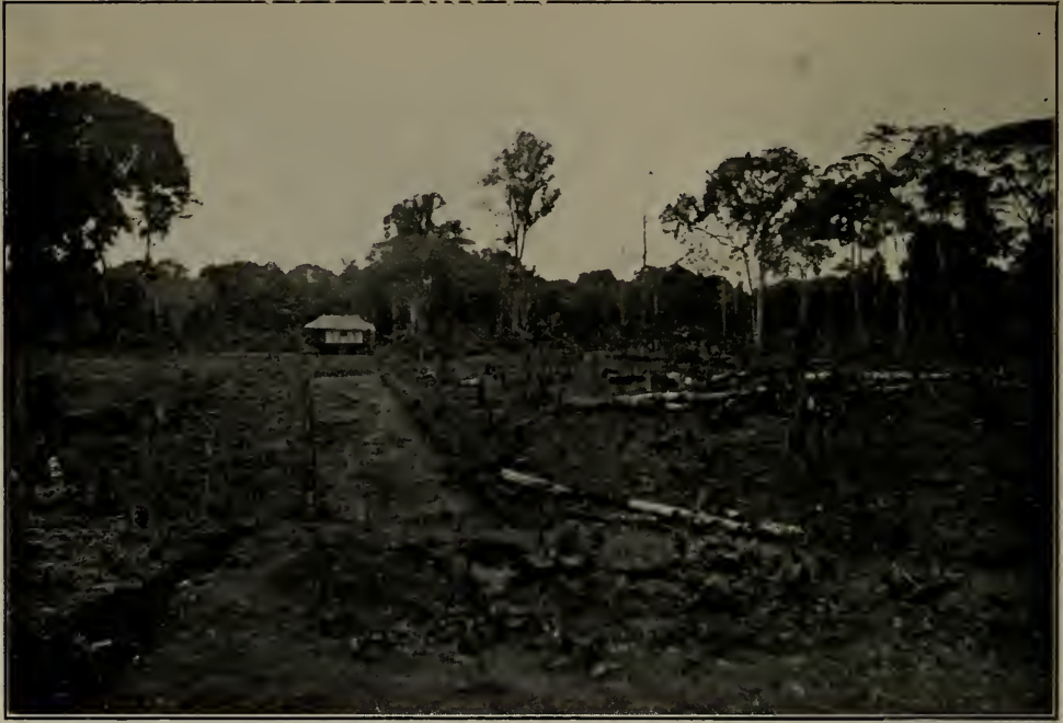
GROUND CLEARED FOR PLANTING.
