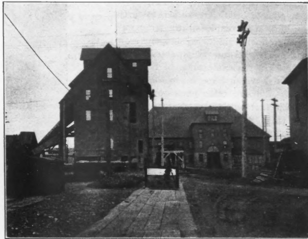
STEEL ROCK HOUSE, MOHAWK SHAFT, NO. 4.
