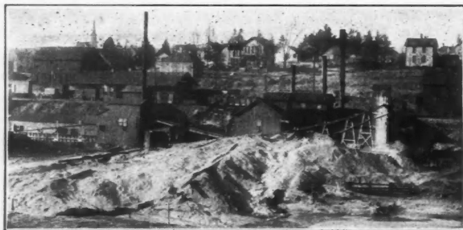
FIG. 1. ENTERPRISE MILL, PLATTEVILLE, WIS.
