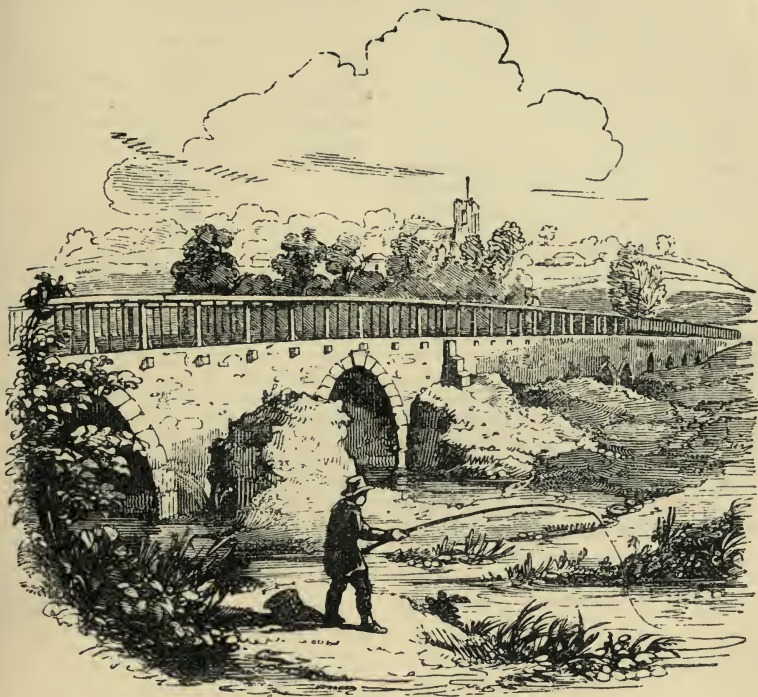
OLNEY BRIDGE, BUCKINGHAMSHIRE.
