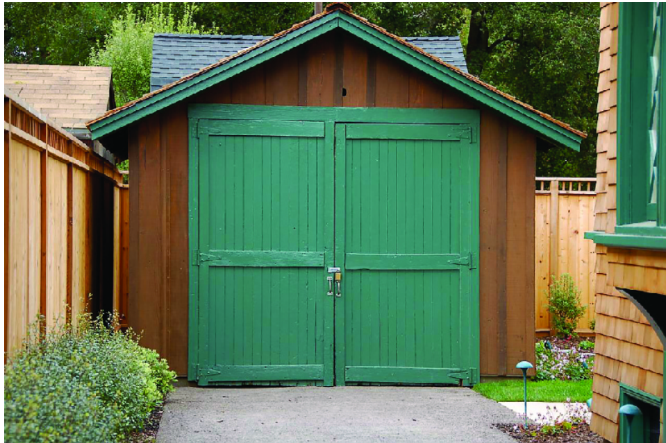
Figure 9.2.2: Hewlett-Packard has restored the original garage in Palo Alto, California, in which its two cofounders, Bill Hewlett and David Packard, former Stanford University classmates, began work in 1938 on the electrical switches and sound oscillators that became their new company's first products. (credit: "HP Garage in Silicon Valley" by "MGA73bot2"/Wikimedia Commons, CC BY 2.0)
