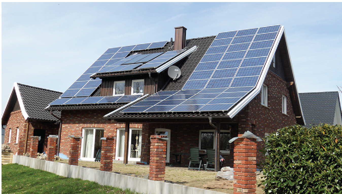
Figure 4.3.9: Although solar panels can reduce your carbon footprint, the tiles are much more expensive than standard roofing tiles. (credit: “Typical Solar Installation” by Tim Fuller/Flickr, CC BY 2.0)
