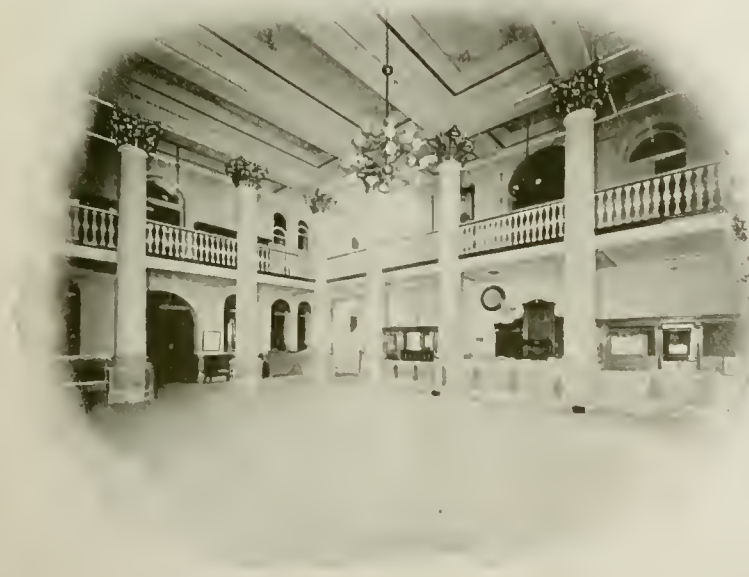
INTERIOR OF THE MAXWELL HOUSE AS IT NOW APPEARS.
