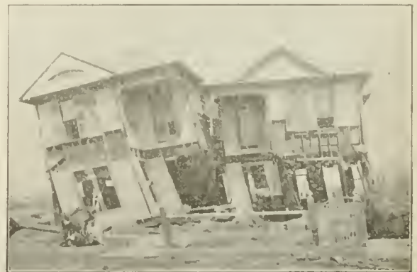
TWIN HOUSES AFTER THE STORM AT GALVESTON.
