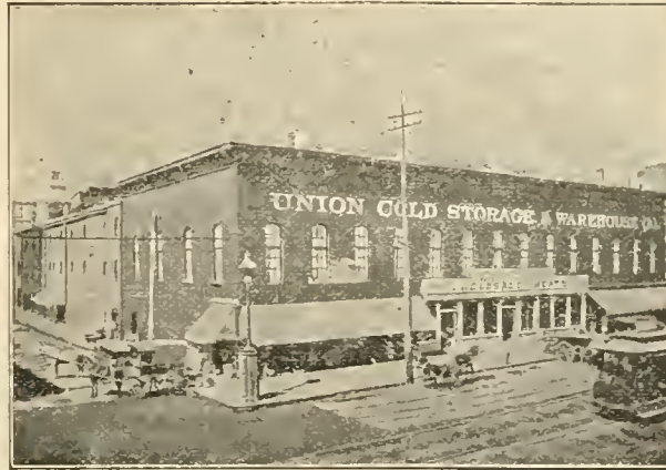
Kalthauslager der Union Cold Storage and Warehouse Company zu Chicago.
