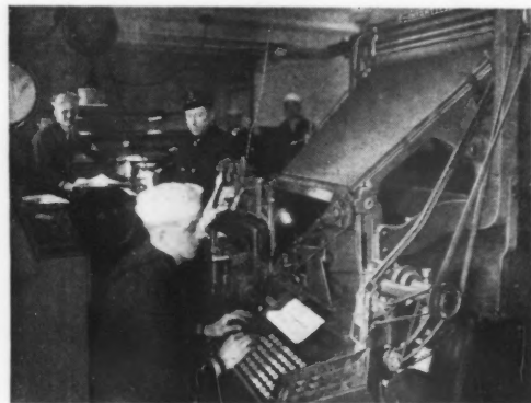
The Leviathan's Intertype as originally installed. It has since been converted into a multiple-magazine machine.
