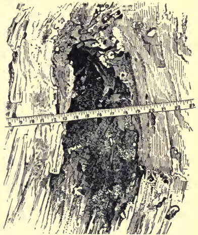
FIG. 120. Inside of the broken limb showing the decay that entered through Fig. 119. The same tree as Fig. 118.
