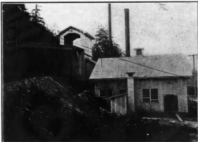
The mine boiler room and compressor plant
