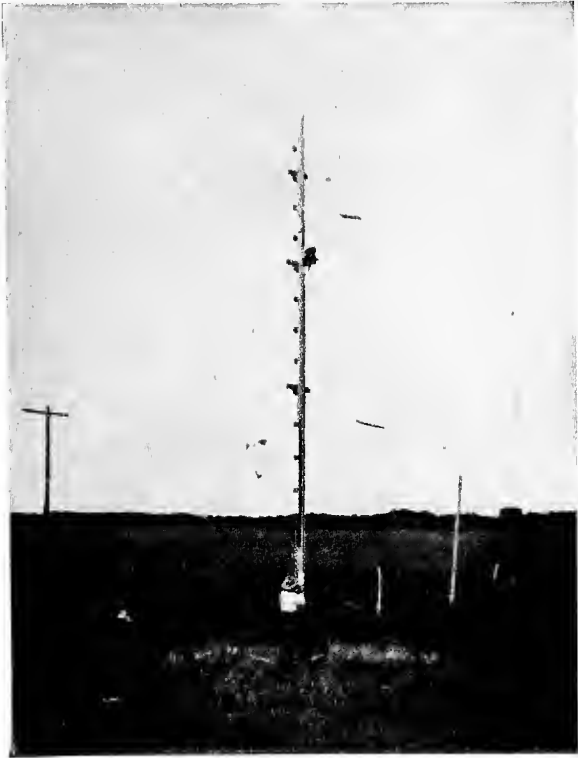
FIG. 96.—Structure for Elevating Signal Lamp over Triangulation Station Used as Mark.
