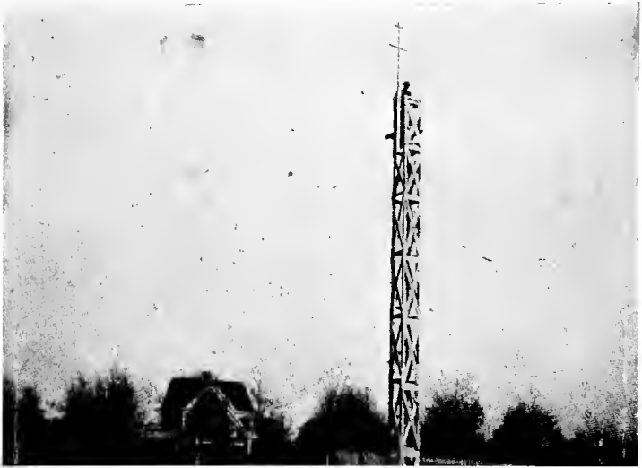
FIG. 97.—Structure for Elevating Signal Lamp over Triangulation Station Used as Mark.
