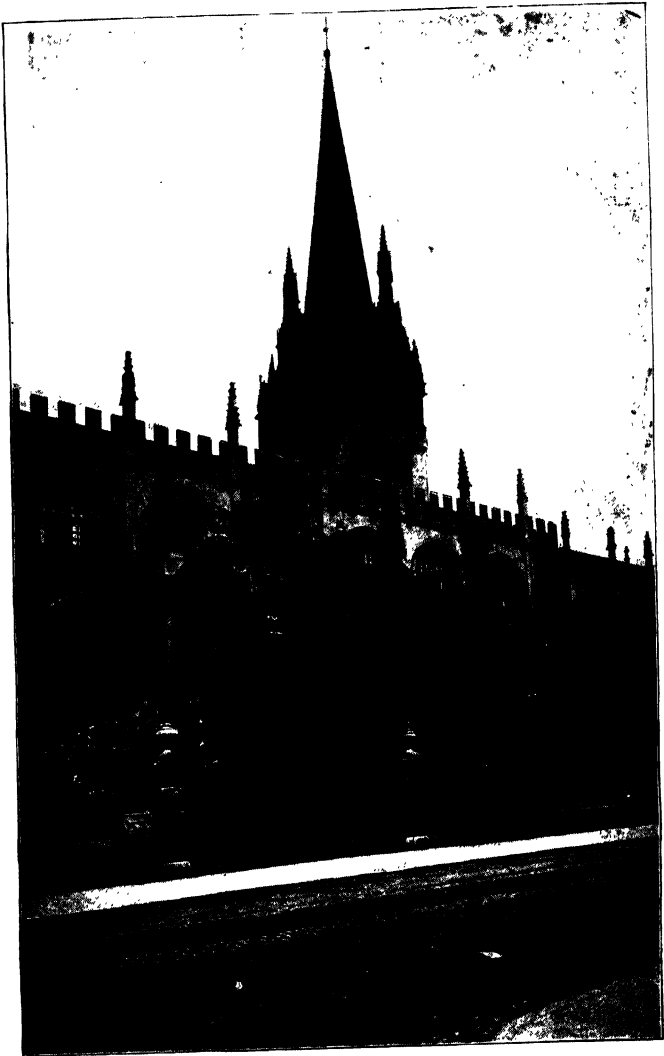
ST. MARY'S, OXFORD. TOWER PARTLY CONTEMPORANEOUS WITH WYCLIF.
