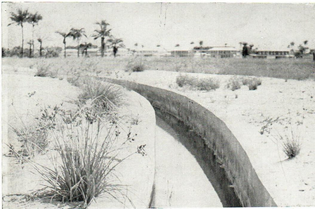
Main drainage outfall, Ikoyi.
