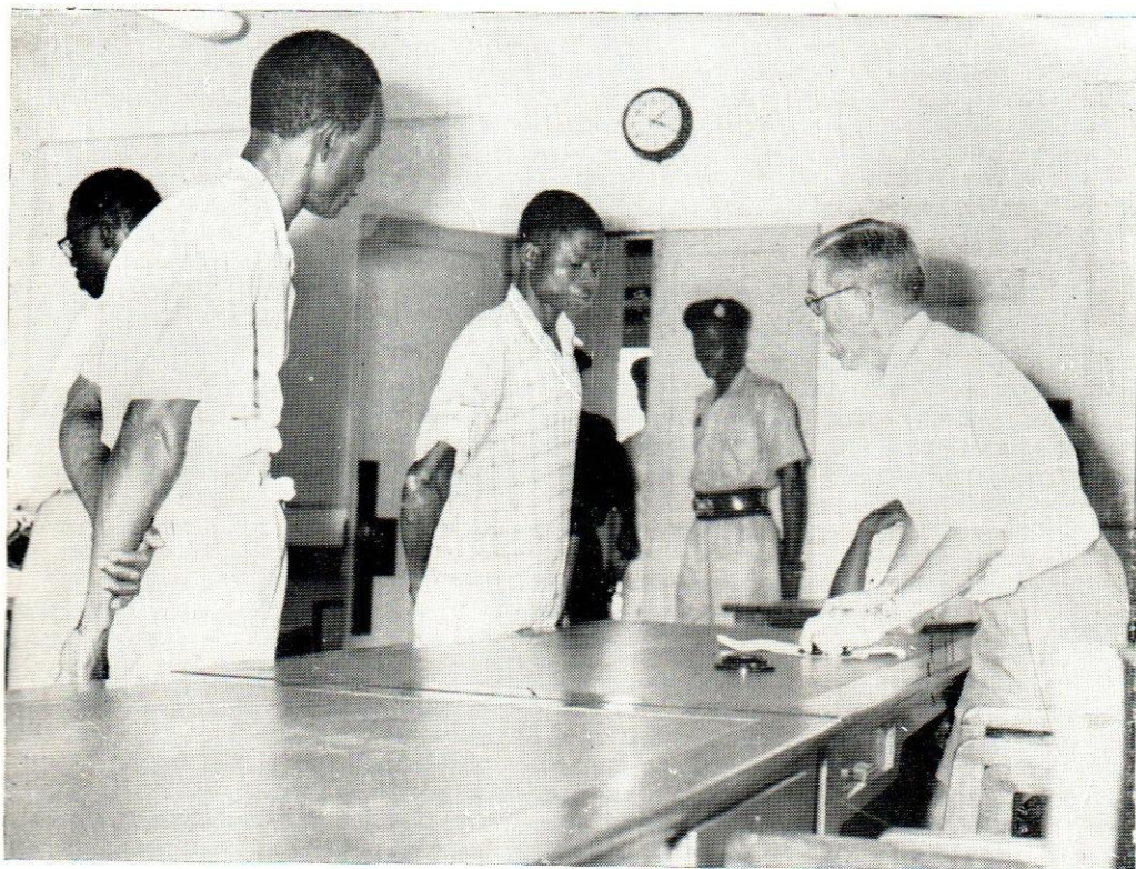
Registration proceeding for Workers' Houses
