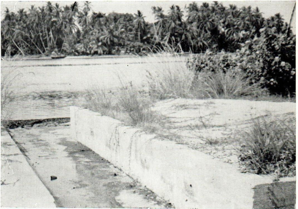
Another view of Ikoyi Main Drainage outfall.
