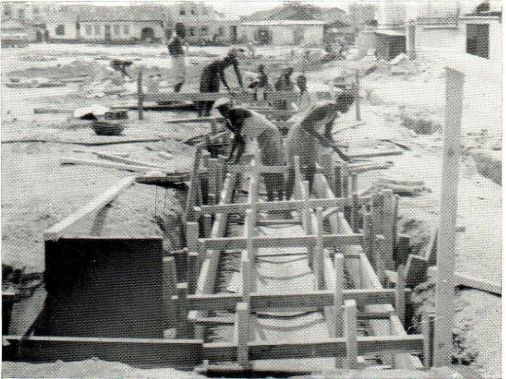
Road and drainage reconstruction in progress on the cleared sites.
