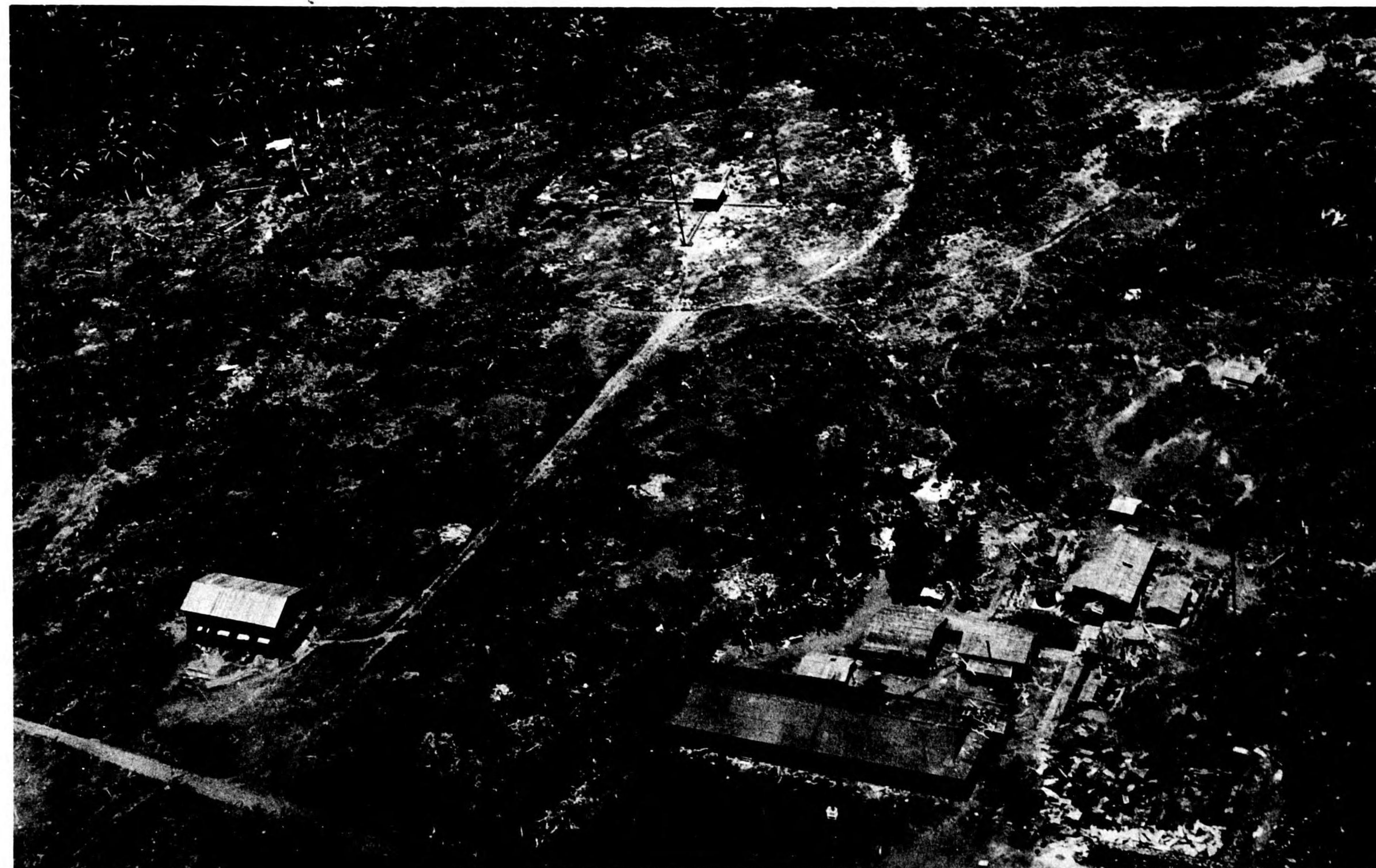
DIRECTION FINDER GENERATOR BLDG. AND CENTER ULALU.
