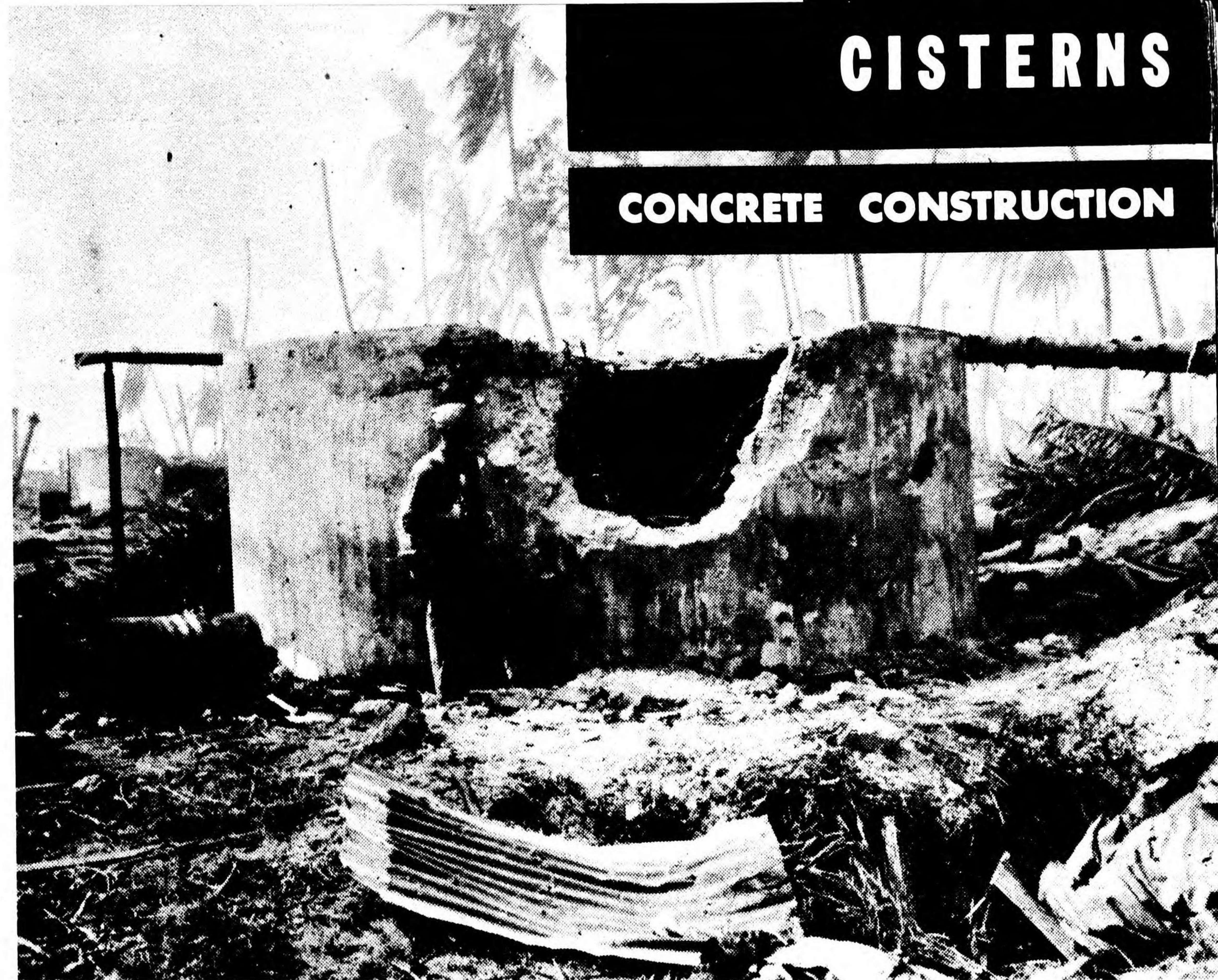
20' DIAMETER CONCRETE CISTERN NAMUR
