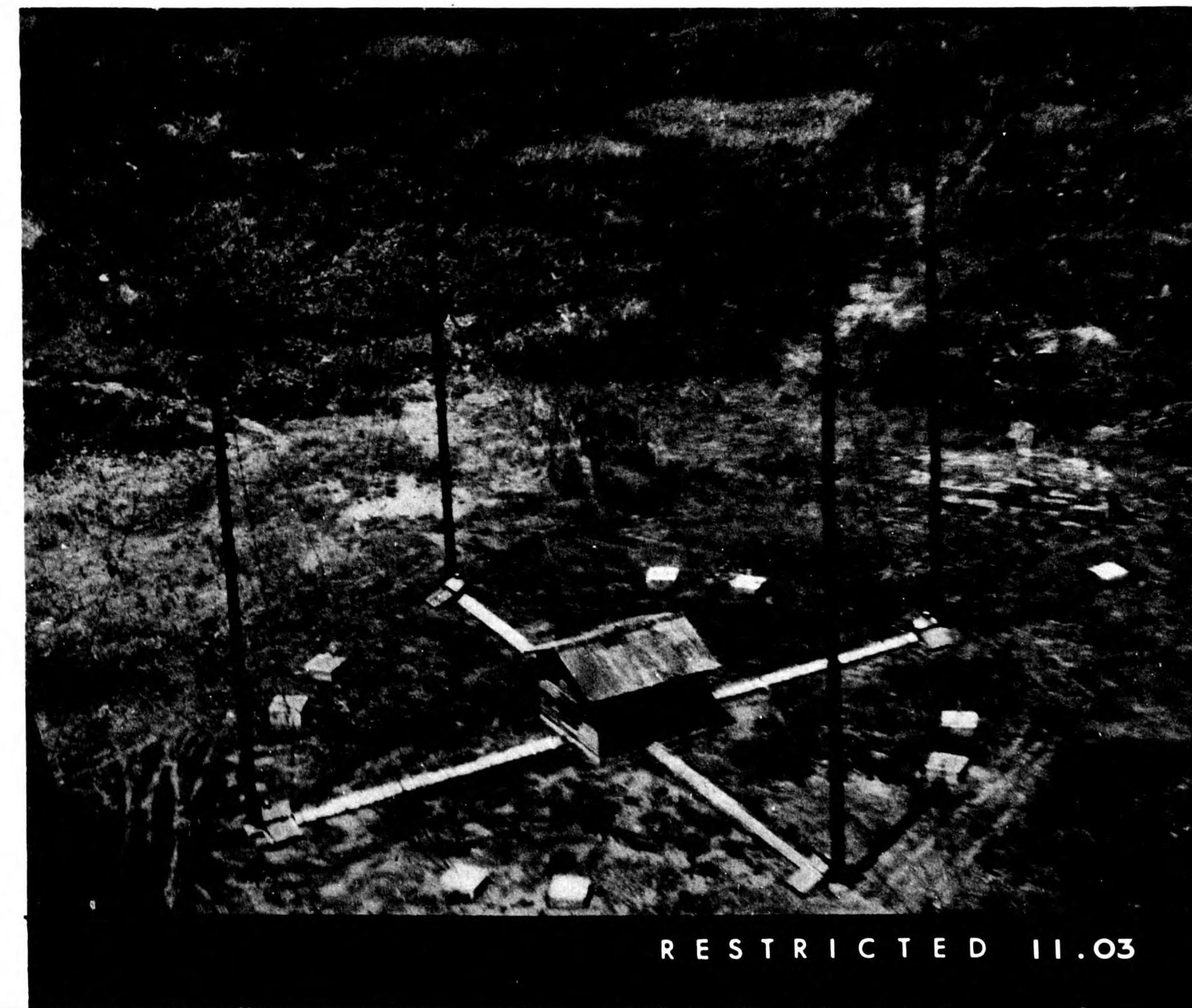
D.F. AND ADCOCK INSTALLATION • RABAU
