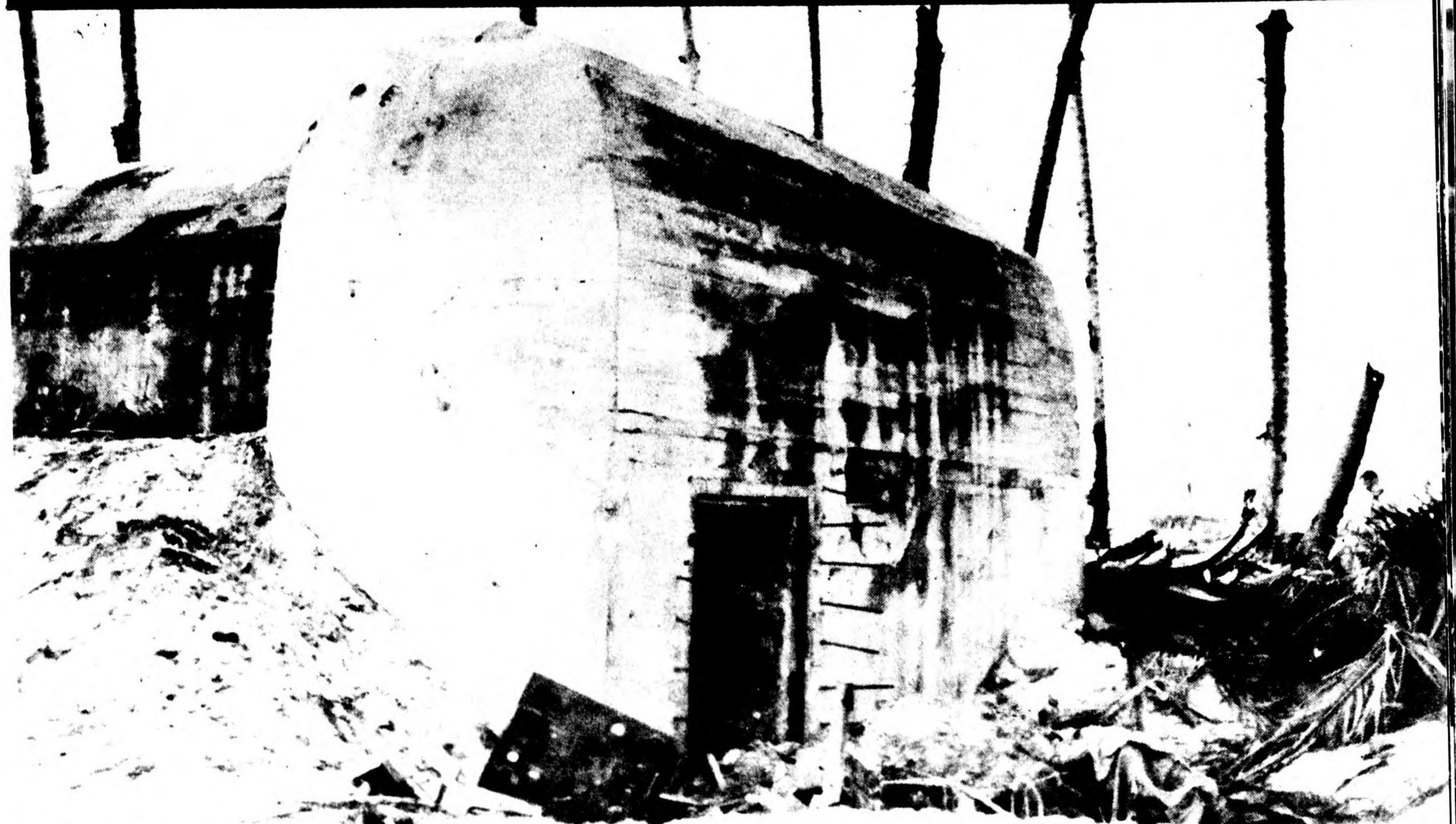
REINFORCED CONCRETE PERSONNEL SHELTER - ROI ISLAND
