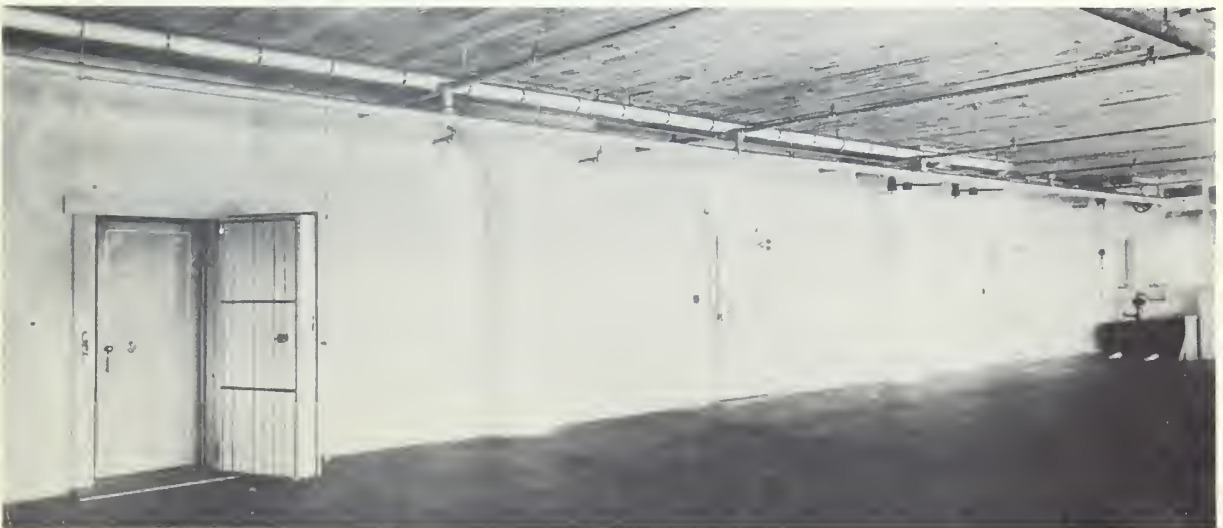
Figure 2.--Battery of three large fumigable fur-storage vaults constructed in a modern concrete building, equipped with devices for regulating temperature and humidity and for introducing and removing the fumigant. The building is also equipped with burglar alarms. At right, on warehouse floor, note storage for fumigant and pump for forcing fumigant to any room desired. These rooms have been operated successfully in southern California for more than 30 years. (Figure 32 of Cir. 369.)
