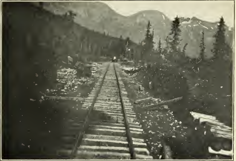
FIG. 1.—VIEW ON ALASKA CENTRAL RAILWAY.
