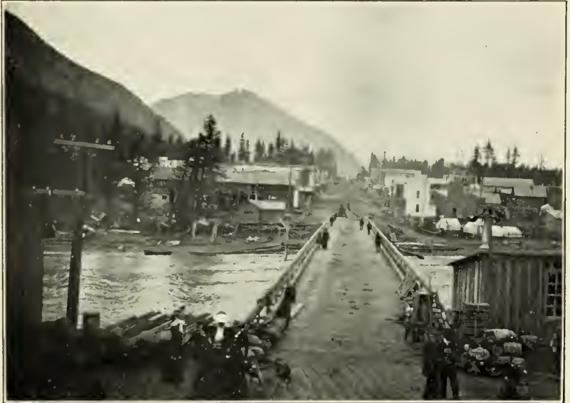
FIG. 2.—TOWN OF SEWARD, RESURRECTION BAY, TERMINUS OF ALASKA CENTRAL RAILWAY.
