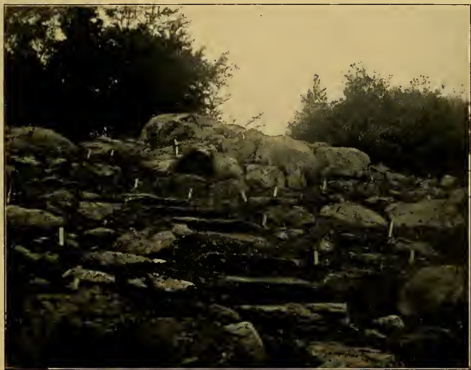
BANK TYPE. (In course of construction.)
