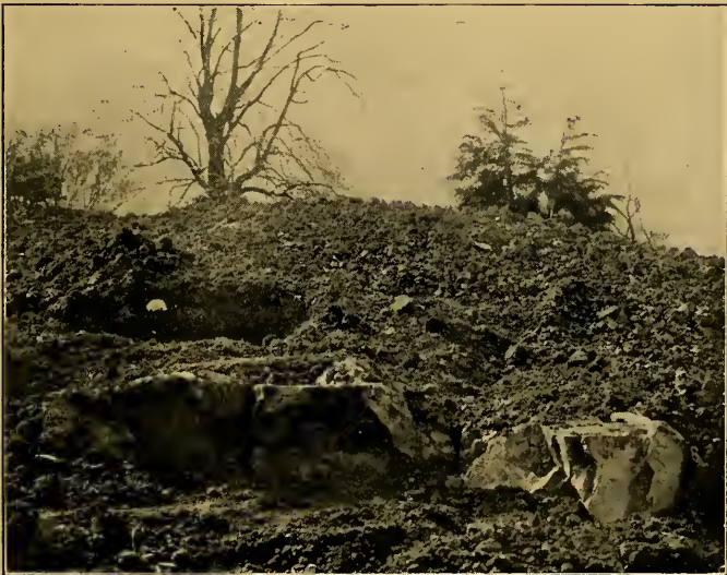
FIRST LINE OF ROCKS LAID.
