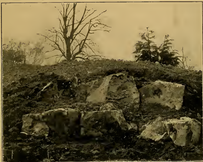
SECOND LINE OF ROCKS IN POSITION.
