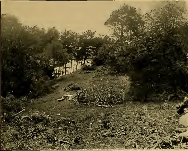
BANK TYPE. (Site being cleared.)
