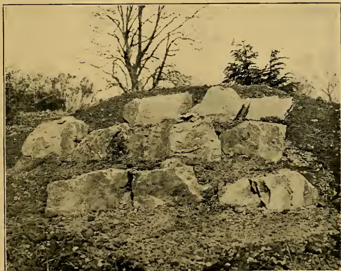
ROCKWORK ADVANCING UP THE HILL.
