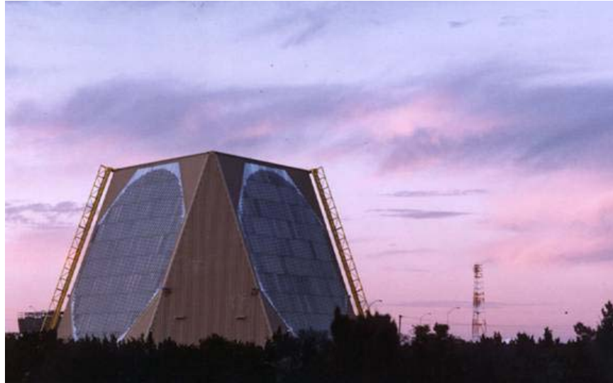
Figure 23 PAVE PAWS UHF, Solid-state, Dual-faced Radar System in Cape Cod Air Force Station, Massachusetts (From Ref. [27]).
